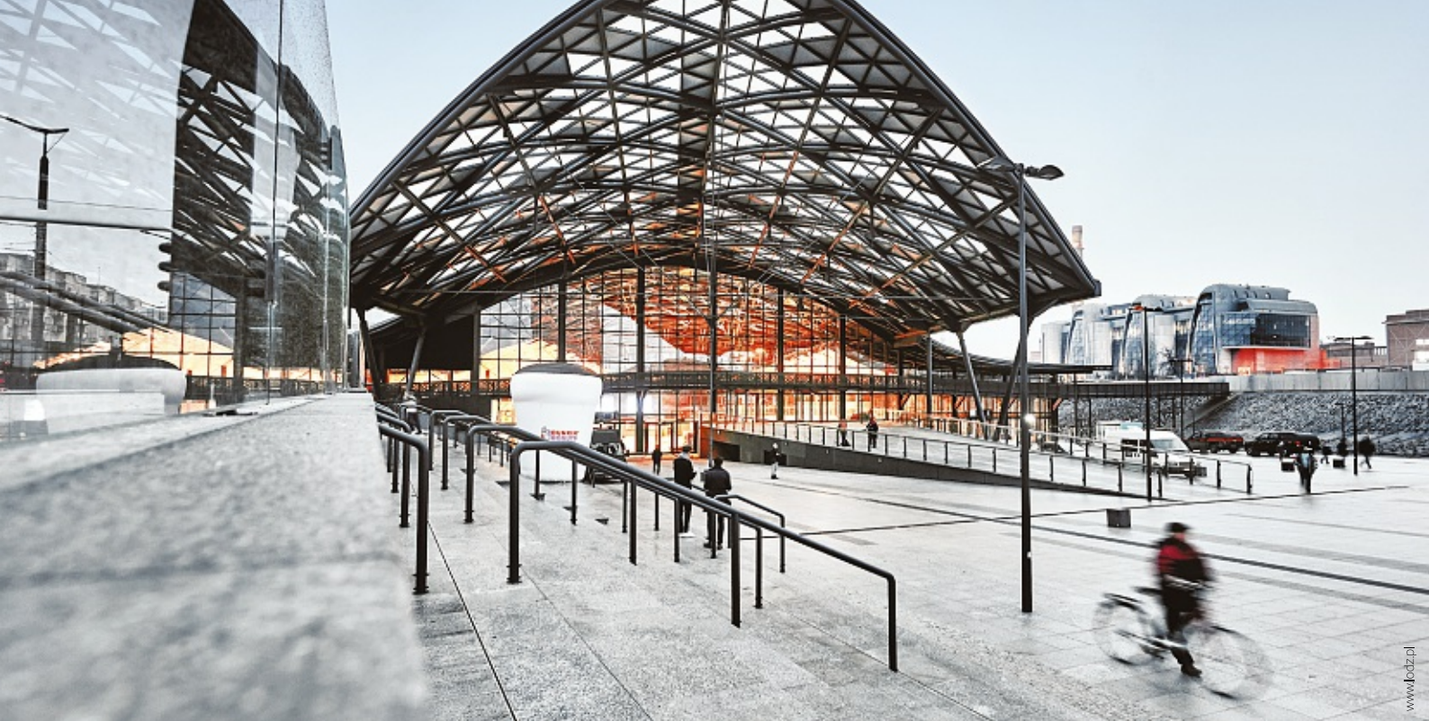
Speedy solution: Łódź Fabryczna station has cut the train time to Warsaw down to 70 minutes
